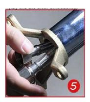
9.Connect the mail body of the tap with the pre-embedded water inlet and tighten the
