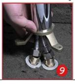
2.Wrap the PTFE tape around the joint and tighten the joint(lay the tile after embedding)
